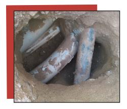
After underground utilities are electronically designated, the next stage in data reliability that is equivalent to Quality Level A, is obtained by Vacuum excavation, also known as, potholing.
